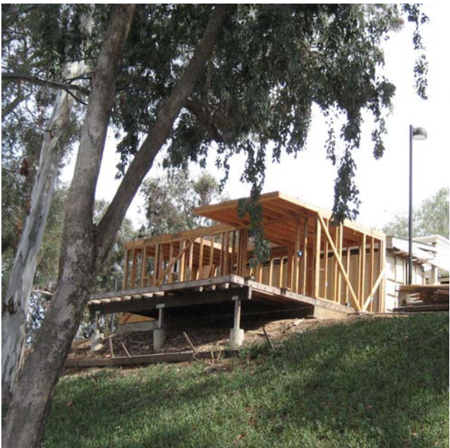
Construction Academy projects at Wake Campus
