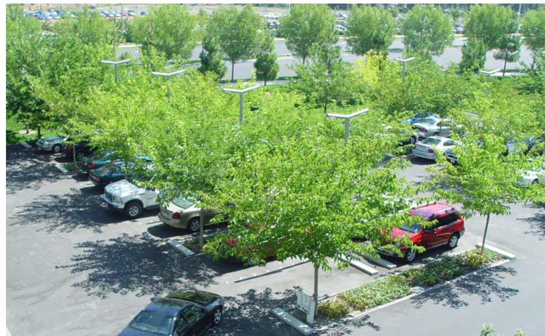
Wide swaths of planting areas break down the expanse of asphalt and increase permeability within the parking lot. Trees provide shade cover and reduce heat island effect.
